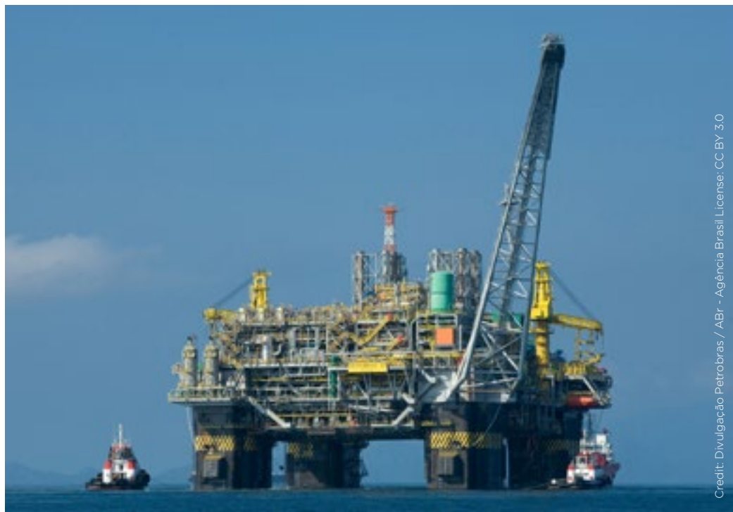
Description: Oil platform P-51 in Brazil
